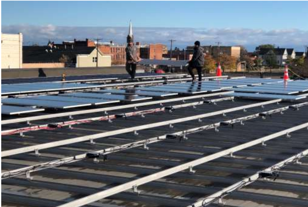
Jolma Electric employees installing solar panels
